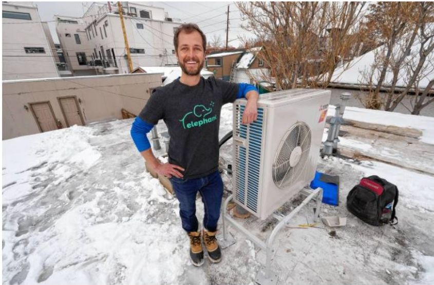
David Richardson, co-founder of Elephant Energy, leans on a condenser placed on the roof during the installation of a heat pump in an 80-year-old rowhouse last January in northwest Denver. AP
